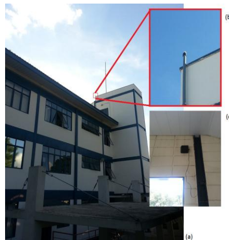
Figure 2: (a) Sensor installed on rooftop; (b) sensor detail; (c) Radio transmitter circuit inside building.
